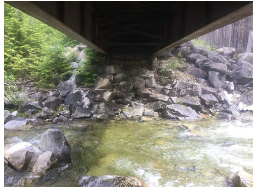
Right Bank Abutment when facing downstream
