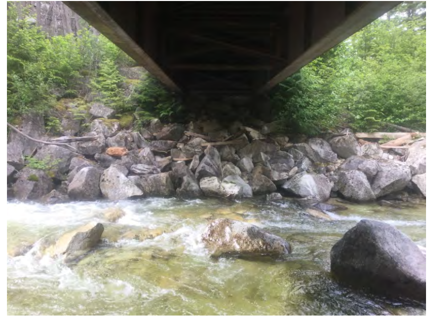
Left Bank Abutment when facing downstream
